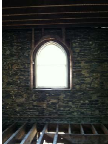
Existing Side windows- clear glazing
