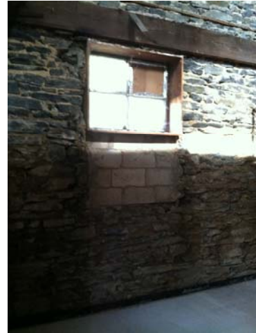
Basement window to be restored to original opening size.
