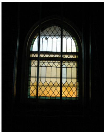
Original stained glass window from Pastor's Office (to be retained by applicant).
