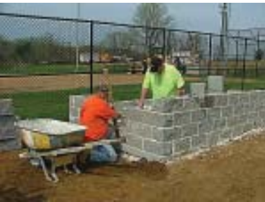
Township forces building dugouts
